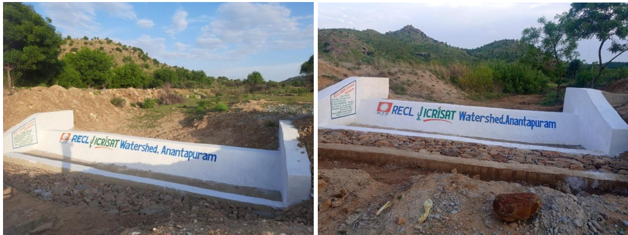
Figure 3. Check dams constructed on the farms of (L) Mr K Siva Sankar in Cherlopalli village and (R) Mrs H Lakshamma in Settipalli village, Anantapur watershed, Andhra Pradesh.
