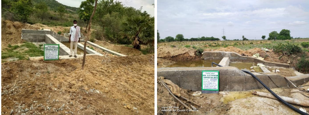
Figure 24. Check dams constructed on the farms of (L) Mr S Kondanna and S Anjaneyulu in Peddagudem village and (R) Mr Ch Ramulu and B Kurumurthy in Kadukuntla village, in Wanaparthy watershed, Telangana.
